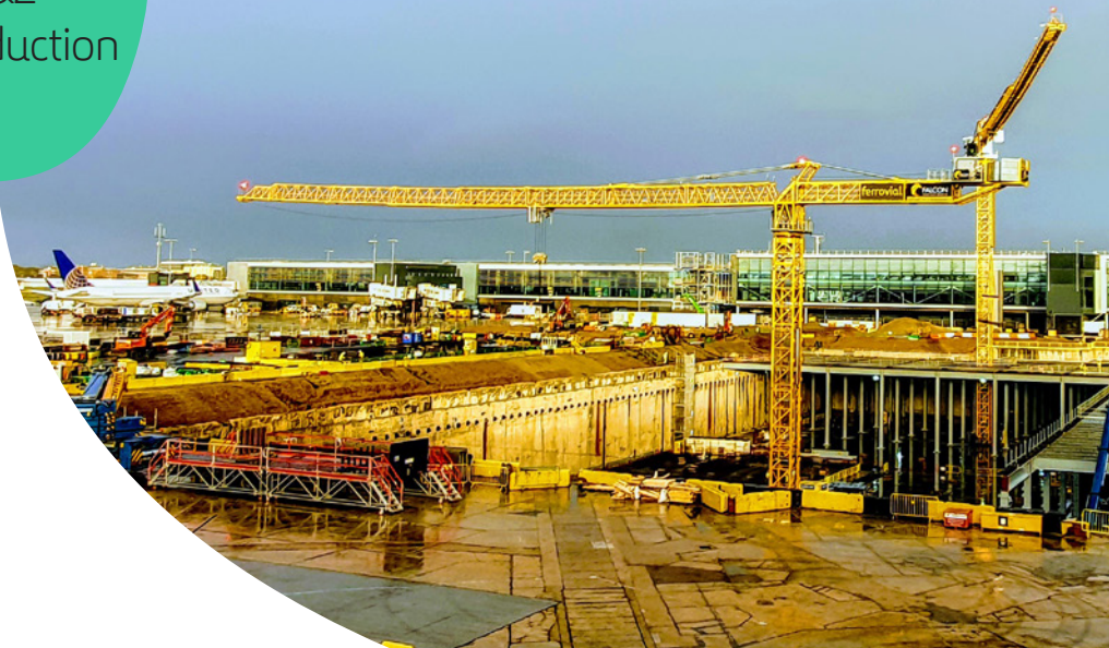
Engineering Progress – Kilo Apron Development Substructure at Heathrow
