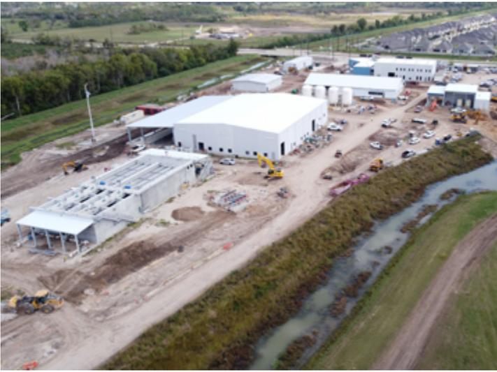
Activated Carbon vessels, these four 27' high by 14' diameter vessels eliminate water odor and taste before chemicals are injected and water is distributed to the final consumer.
