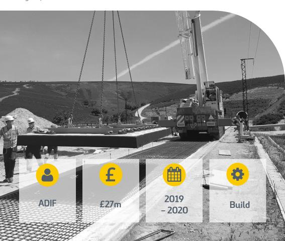
The construction of the high-speed rail track from Pedralba – Campobecceros was just over 81km consisting of three construction methods; 63km through slab track, concreted in situ, 19km ballast track with mono-block sleepers, and 2km pre-cast slab track. This is due to the geographically complex area which meant 61km of the track was located in 10 tunnels and on 4km of viaducts.
