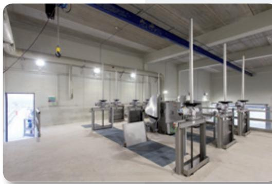
Subsequent to arriving at the plant, the water is sent to the three filtering channels, two of which are fitted with automatic fine screens. The third filtering channel functions as a bypass line and is equipped with a manual bar screen with a space between bars of 20 mm.
