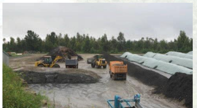
Landfill and Tecnosols' extension
