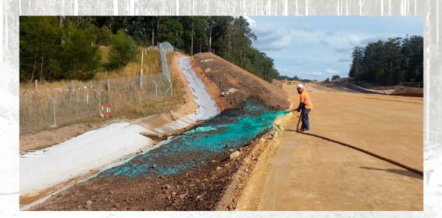
The Warrell Creek to Nambucca Heads Project requires environmental best practice in terms of erosion and sediment control during the construction phase of the project, enabling Pacifico to meet its Environmental Protection Licence requirements. In order to achieve this large quantities of geotextile and similar products are required to provide temporary stablisation and erosion protection during construction.
